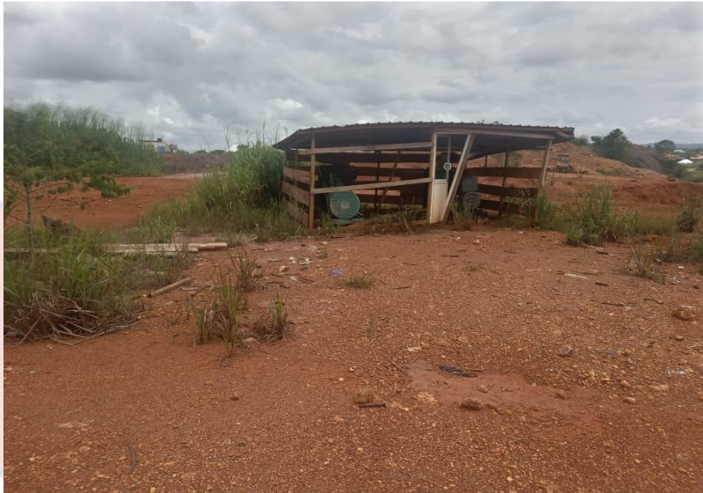
Plate 7: An abandoned water plant at a site at Akwaboso
