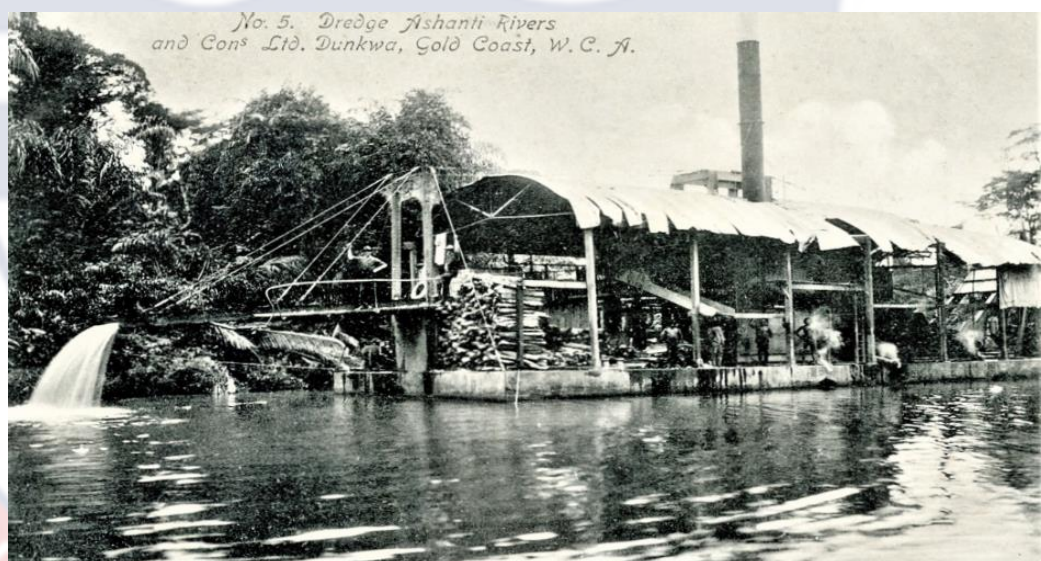
Plate 2 A dredging machine in Offin River at Dunkwa
