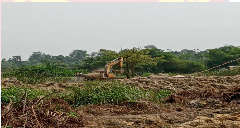
Plate 5: Excavator at a site at Diaso
